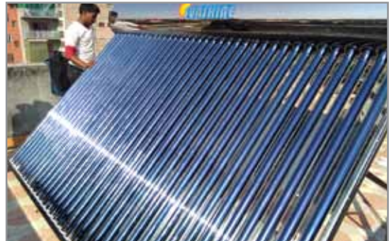
Installing Solar water heater in Orphanage
